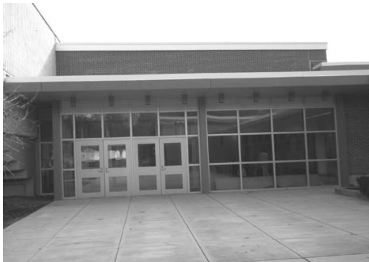
Students are encouraged to exit through the old main entrance during a fire alarm, which had been inaccessible during the prior phase of the construction project.
